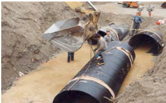
1994 Culvert Installation (photo credit: M. Foy)
