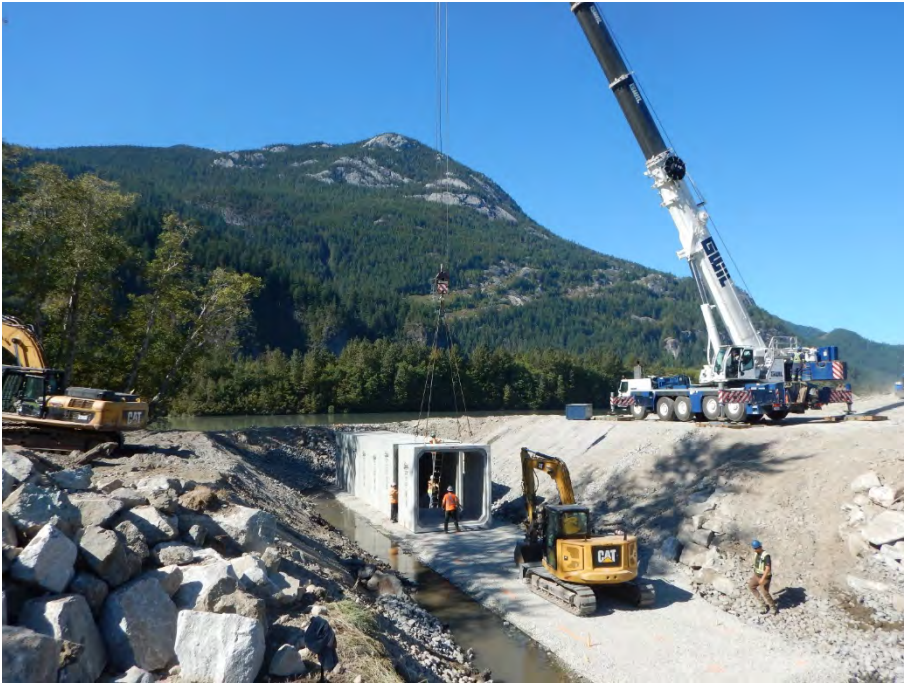
September 10, 2020 culvert segment placement with Gwil 300-t crane
