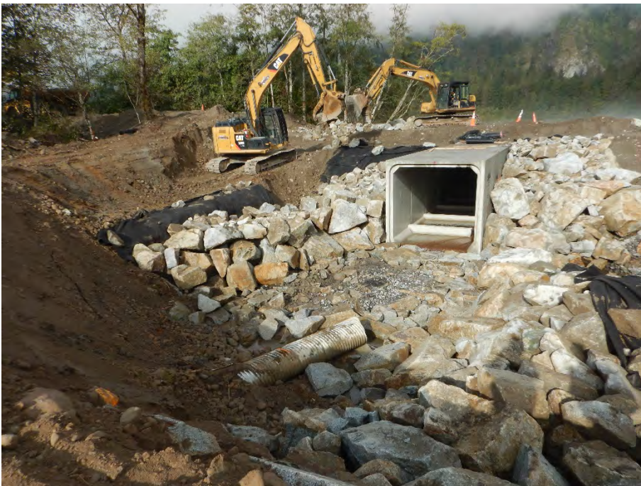
September 22, 2020 backfilling; note geotextile layer below armouring
