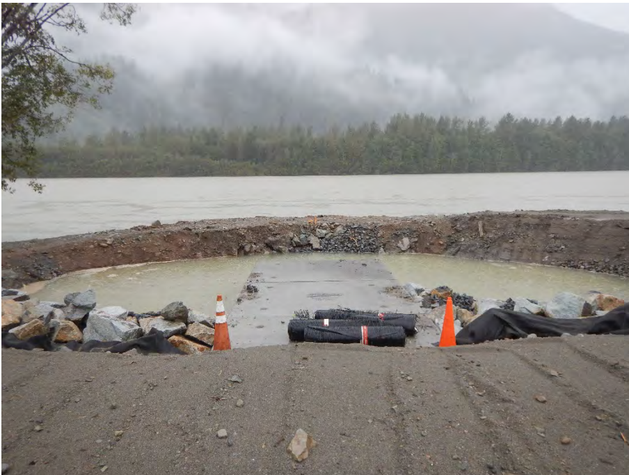
September 23, 2020 reconstructed river coffer dam during large high-water event able to keep out floodwaters
