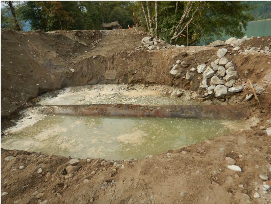
Photo taken September 1 showing the exposed former 1.2 m steel pipe culvert
