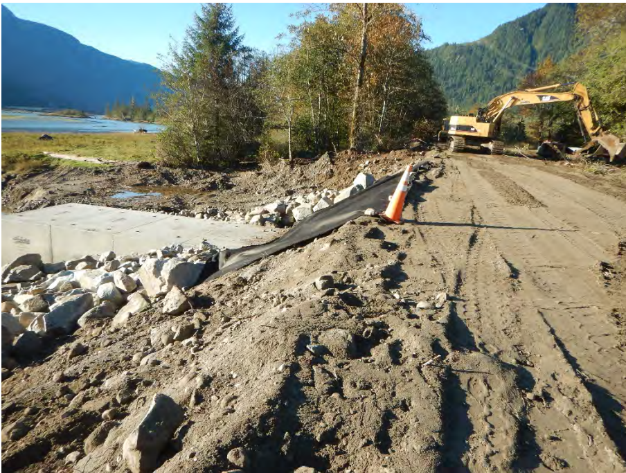
September 29, 2020 geofabric placement on estuary side (above photo) and river side (photo below)
