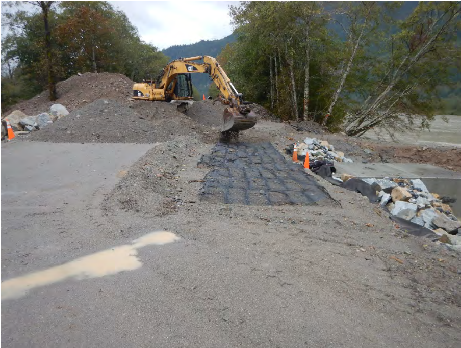
September 24, 2020 placement of geogrid to prevent road slippage
